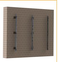
Apply T1 profiles to the vertical structure of the building.
