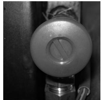
**Safety valve:** this valve acts to prevent over pressurization of the hydraulic system. If the pressure of the boiler or plant exceeds 2,5 bar it drains the water from the circuit.
