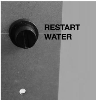
**Safety thermostat with manual reset for the water temperature:** if the temperature of the water tank exceeds the preset safety level of 100 °C immediately stops the operation of the boiler and the display will show **"ALAR-SIC-FAIL"**. To restart you need to reset manually.
